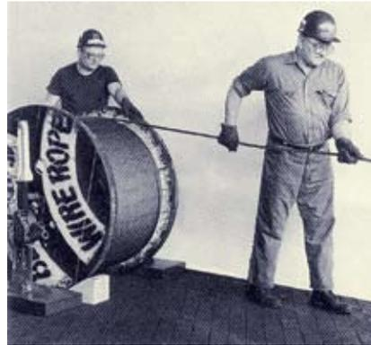
**The Wrong Way To Unreel.** If a reel of wire rope is laid on its flange with its axis vertical to the floor and the rope unreeled by throwing off the turns, spirals will occur and kinks are likely to form in the rope. Wire rope should always be handled in a way that neither twists nor unlays it. If handled in a careless manner, reverse bends and kinks can easily occur.
