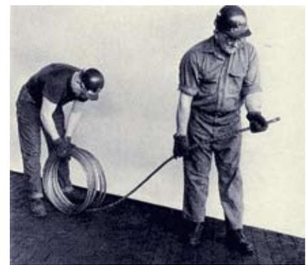
**The Wrong Way To Uncoil.** If a coil of wire rope is laid flat on the floor and uncoiled by pulling it straight off, spirals will occur and kinking is likely. Torsions are put into the rope by every loop that is pulled off, and the rope becomes twisted and unmanageable. Also, wire rope cannot be uncoiled like fiber rope. Pulling one end through the middle of the coil will only result in kinking.
